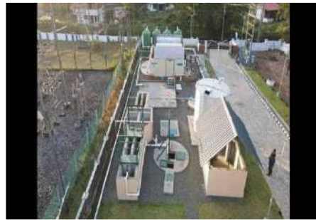
1 MLD CSTP at Padanappalam, Kannur
